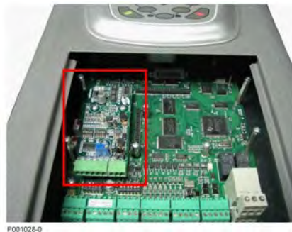
Figure 115: Encoder board fastened to its slot
